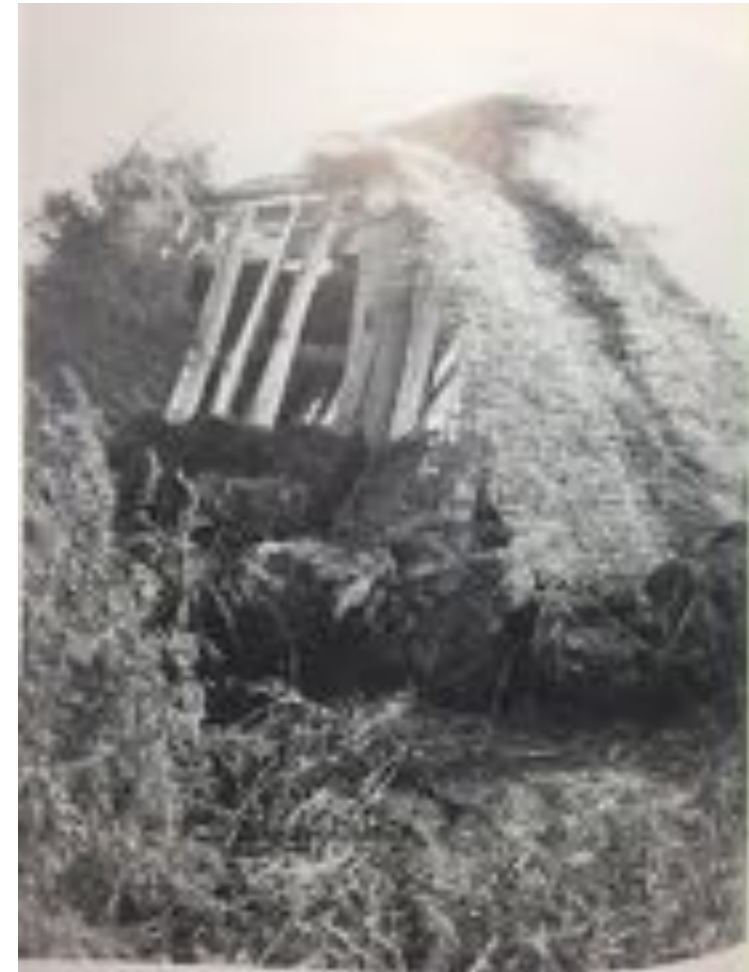
Qasgi construction, showing clearly how grass mats were laid over the wooden frame. Martin Family Collection.
